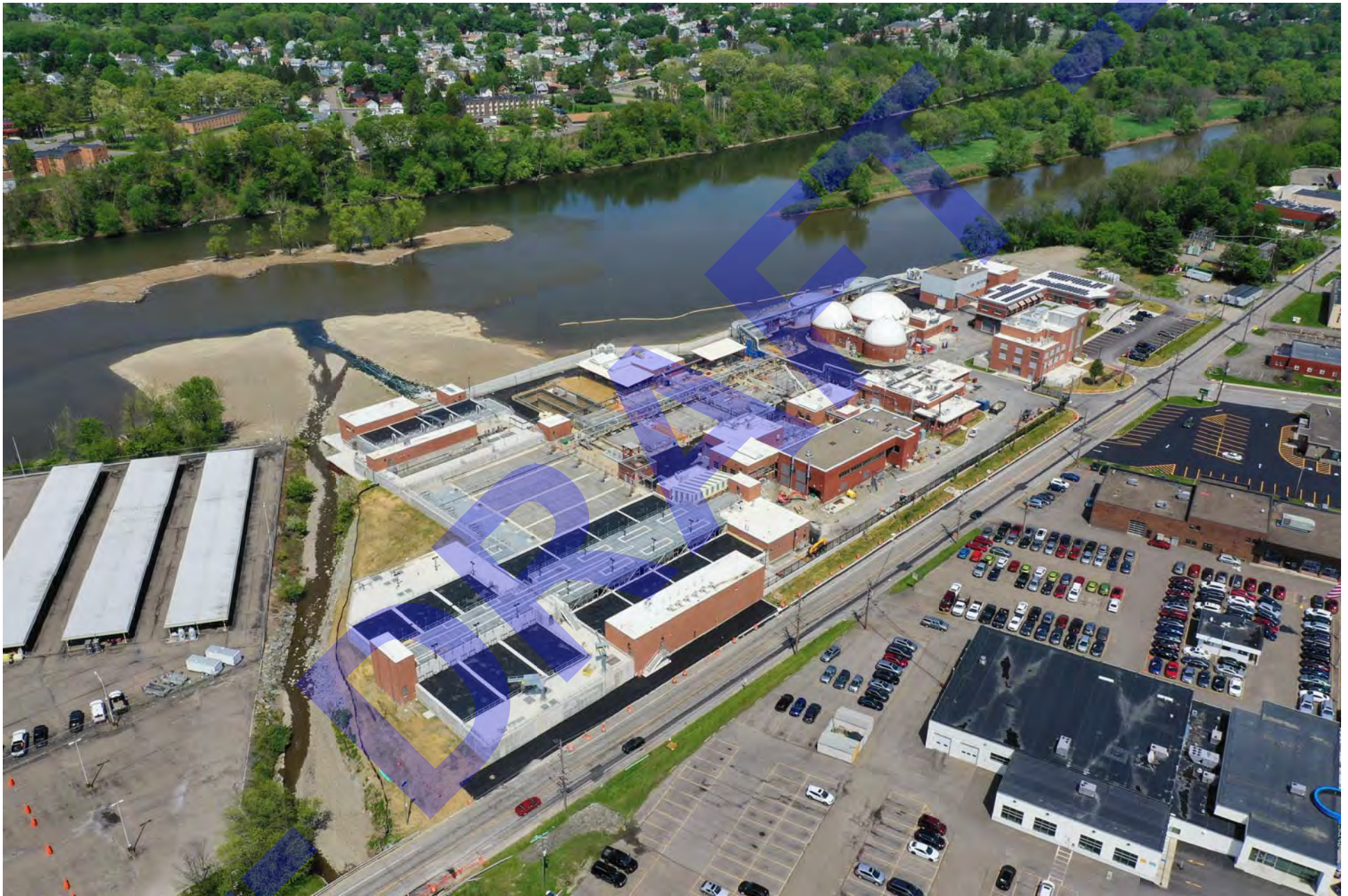
05/25/2020 @ 2:50pm - aerial view from southwest of the Joint Sewage Treatment Plant (construction progress photograph)
