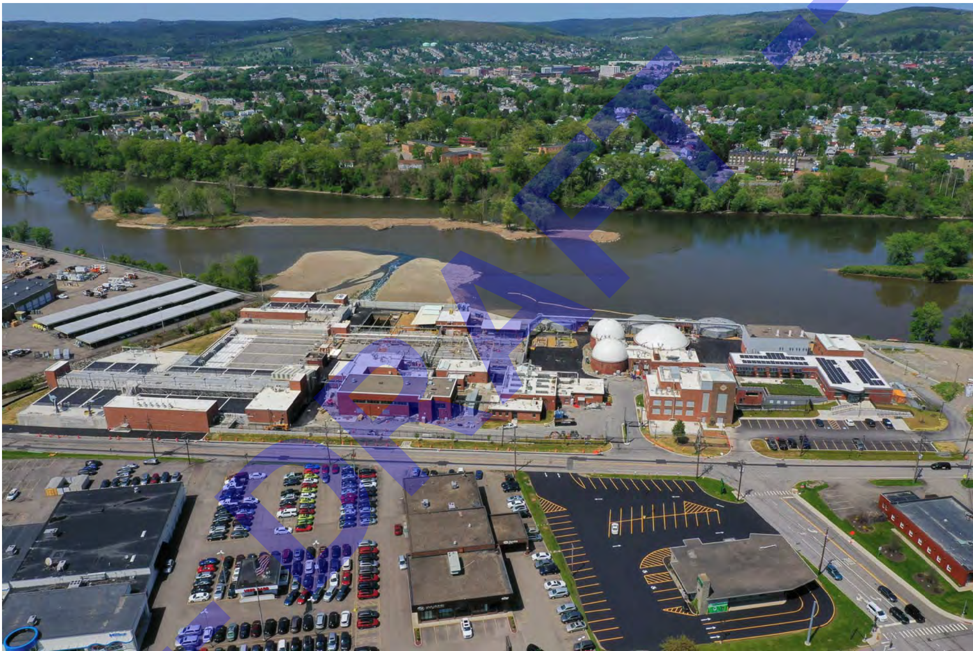
05/25/2020 @ 2:46pm - aerial view from south of the Joint Sewage Treatment Plant with islands in the Susquehanna River connected under a NYS-DEC grant-assisted Joint Sewage Board Water Quality Improvement Project (WQIP). The Village of Johnson City is across the river (construction progress photograph)
