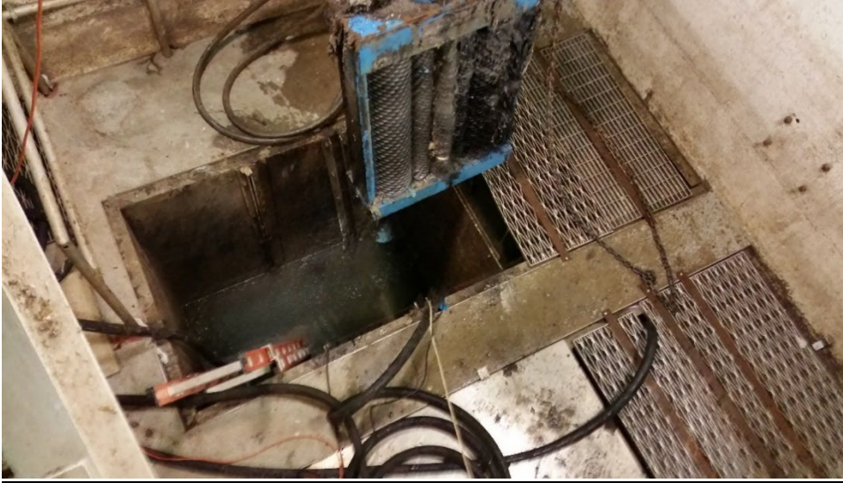
Channel Grinder being removed from West Channel at Terminal Pump Station (TPS)
