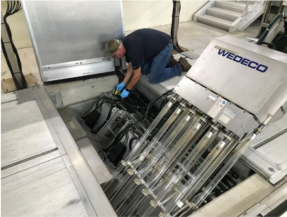
Instrument technician testing position switch. 9/13/2021
